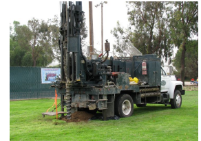
Continuous Core Drill Rig
