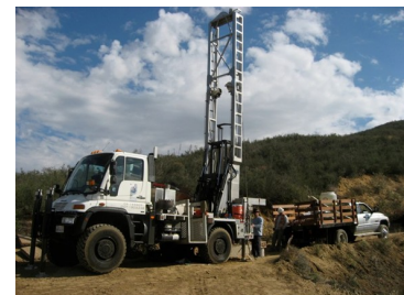
Rotary Wash Drill Rig
