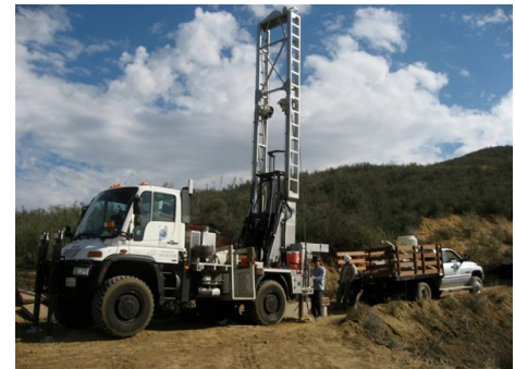
Rotary Wash Drill Rig
