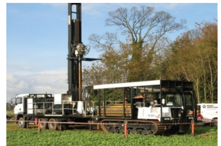
Sonic Core Drill Rig
