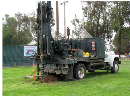
Continuous Core Drill Rig
