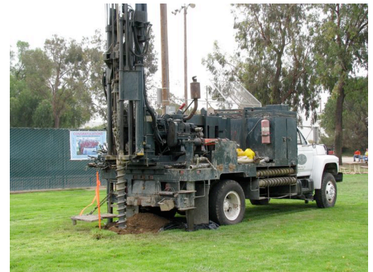
Continuous Core Drill Rig
