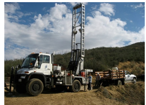
Rotary Wash Drill Rig
