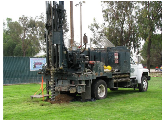
Continuous Core Drill Rig
