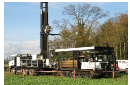
Sonic Core Drill Rig
