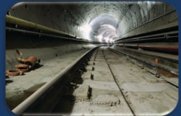
Gold Line Eastside Extension Tunnel
