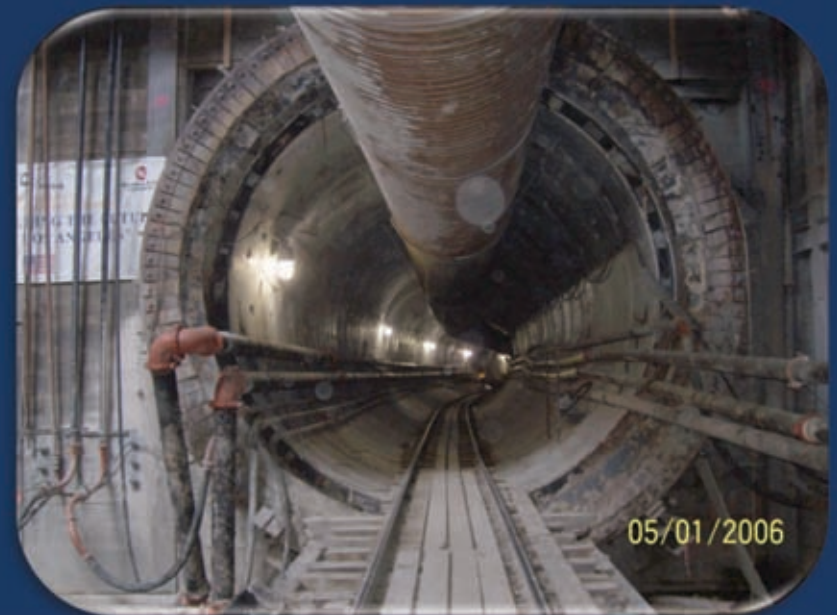
TBM maintains pressure in surrounding earth as it tunnels
