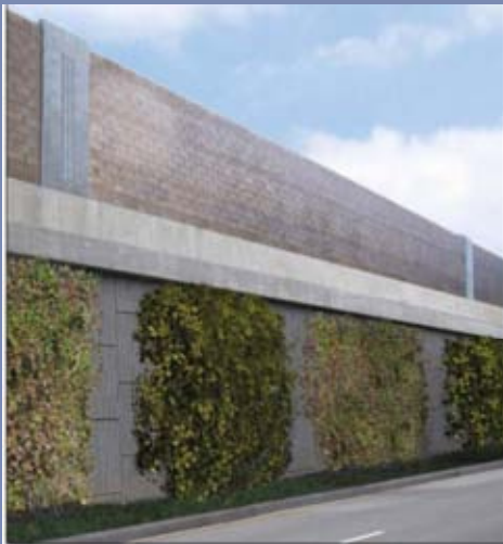
MSE retaining wall with sound wall and pilasters
