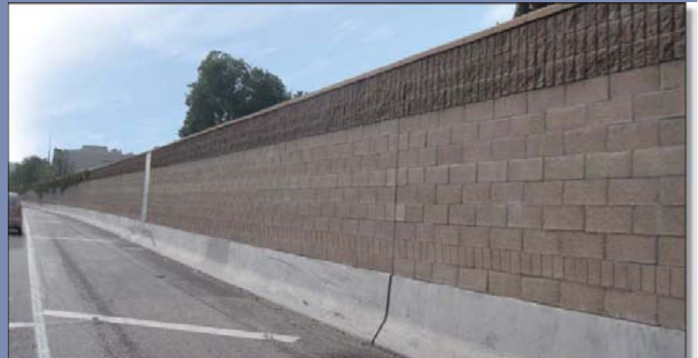
Sound wall at north end of project
