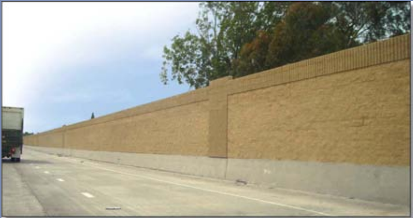
Sound wall at south end of project
