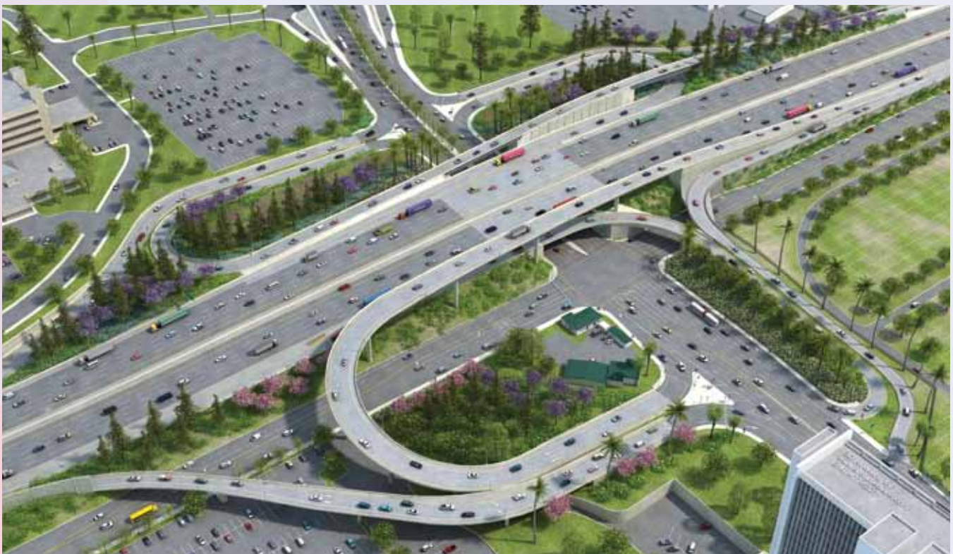
Completed Wilshire Loops (Looking North-West)
