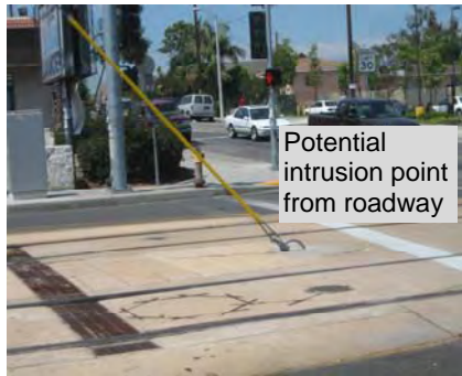
Figure 3 – Unprotected Guy Wire
