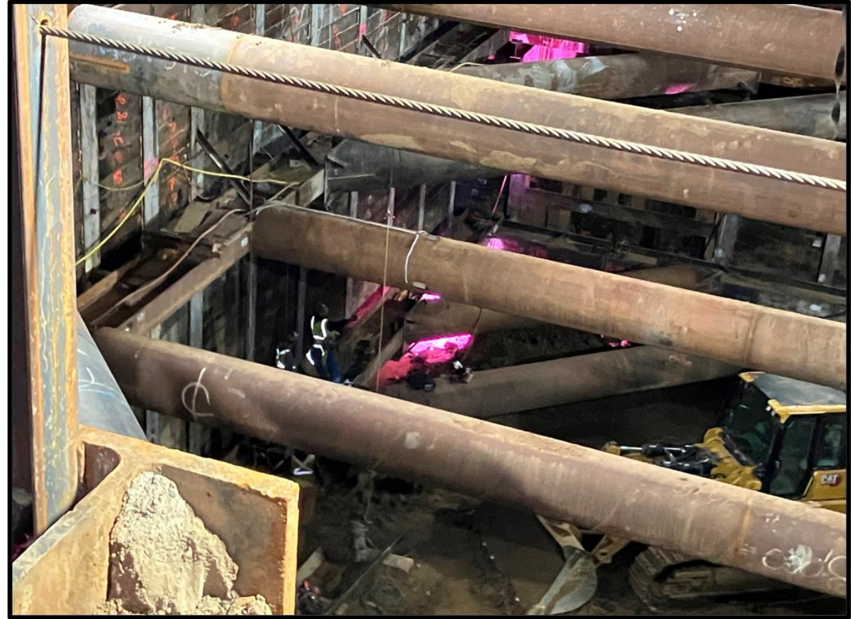
Northeast entrance diagonal struts support excavation.
