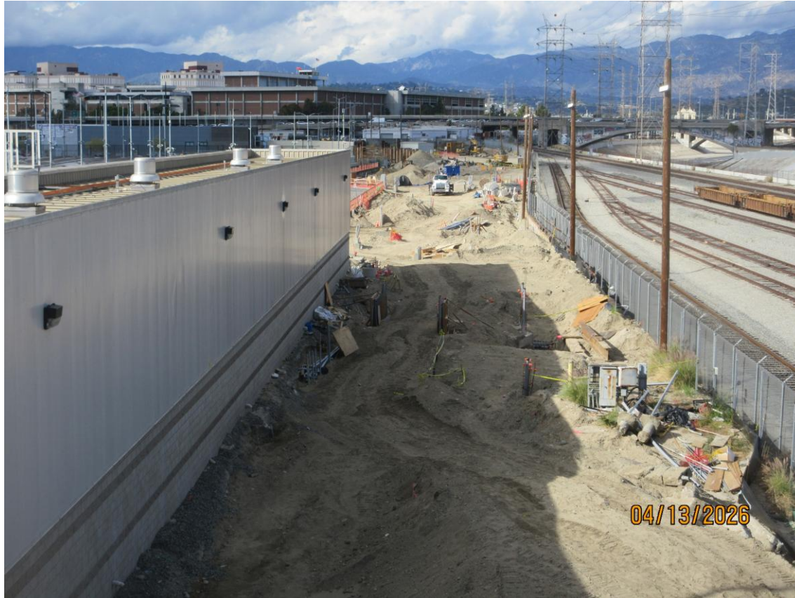
Underground utilities excavation including train control, traction power, and communications (looking North)
