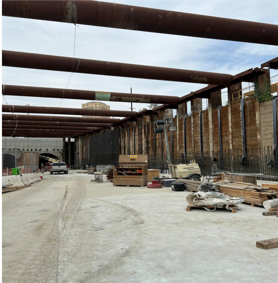
Portal Invert construction and wall construction looking south
