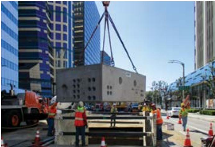
Before station construction can begin, numerous utilities that run under Wilshire Bl, such as water, power and telecommunications, need to be relocated so that service continues while the subway is being built. The image shows Metro contractors lowering a new utility vault into the ground on Wilshire Bl near Westwood Bl.
