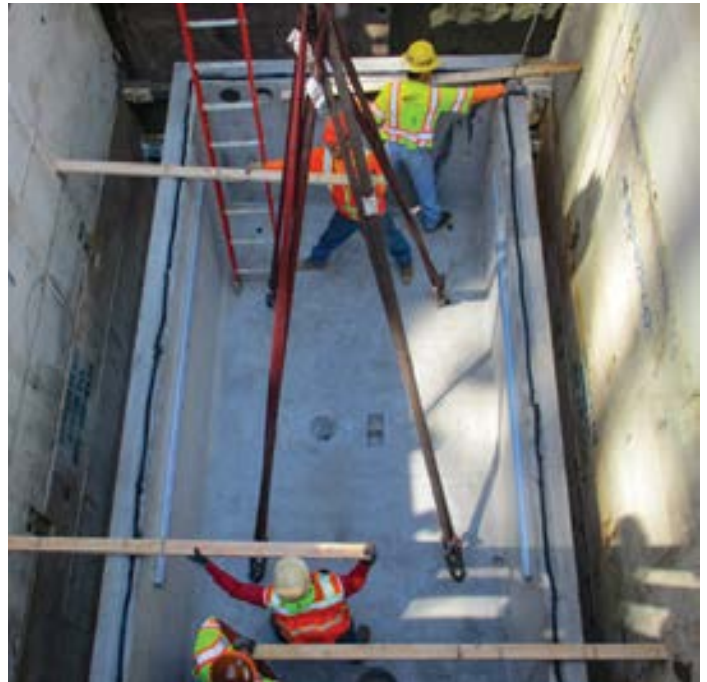
A utility vault is an underground room that provides workers access to utility equipment for maintenance. The image shows Metro contractors installing the new utility vault under the street surface.
