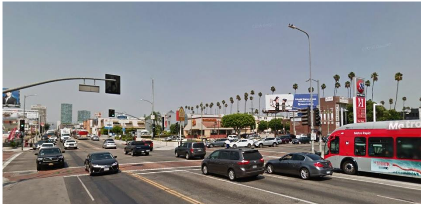
Figure12: Narrow ROW and poor LOS at Vermont Avenue and Olympic Boulevard (facing northbound)
