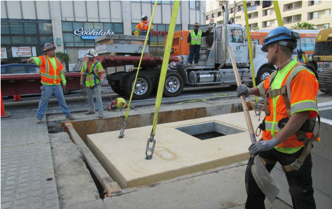
LADWP Power Vault 677 Upper Section Being Installed
